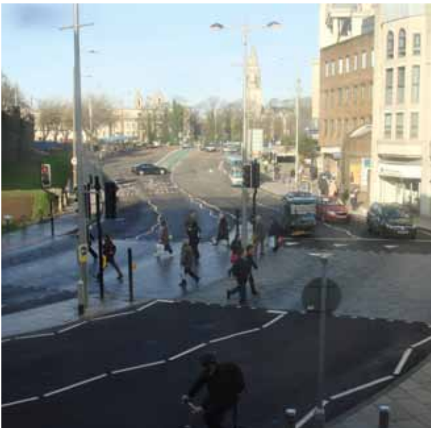
▲ RECENTLY UPGRADED JUNCTION OF KINGSWAY/ DUKE STREET
