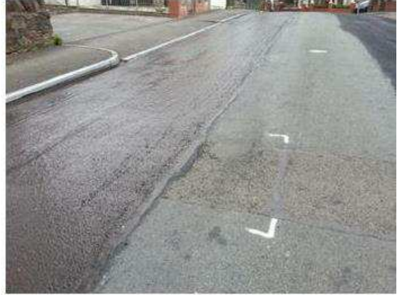
Image 2: Newly laid micro asphalt treatment
