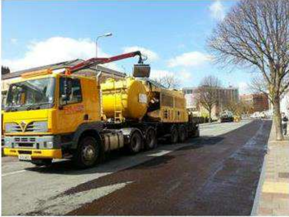
Image 1: Micro asphalt application process
