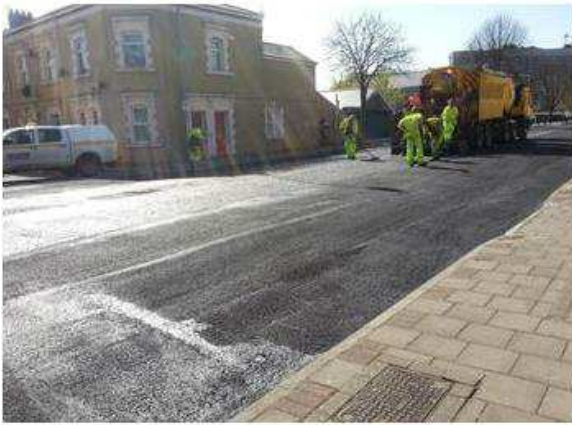
Image 3: Micro asphalt application process
