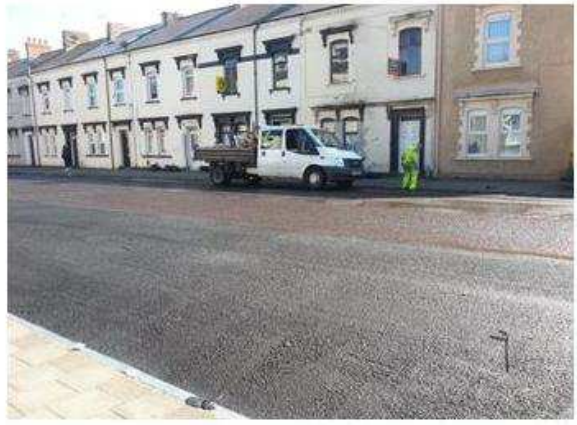
Image 4: Completed micro asphalt treatment process
