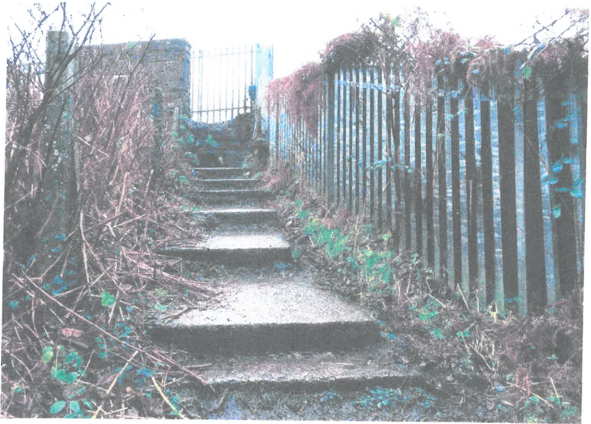
Figure 3: Steep, uneven & slanting steps to access footbridge over
