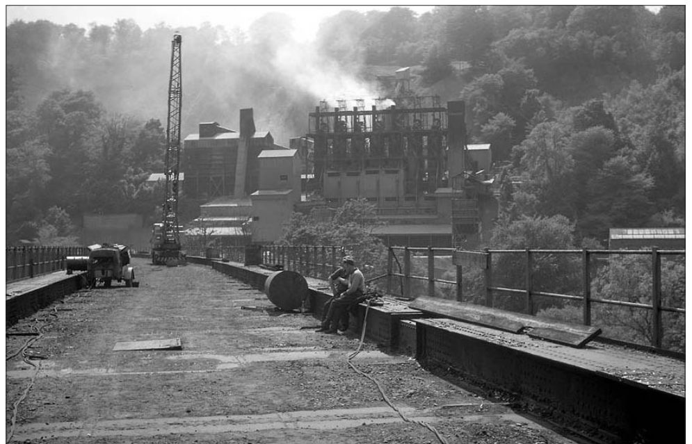
Radyr and Morganstown 50 years ago. A photograph of the Barry line viaduct while it was being demolished c. 1963. Notice the works in the background on the Morganstown side of the gorge, long since gone and the scar has healed.
